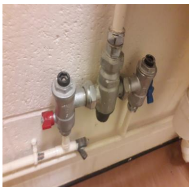
Example of TMV's located within the toilets
