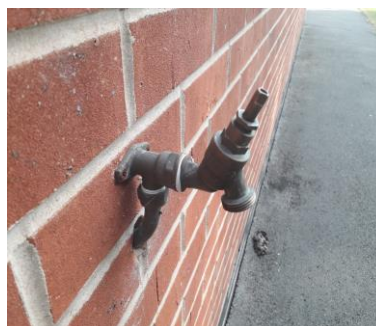
Outside bib tap fitted with no backflow protection
