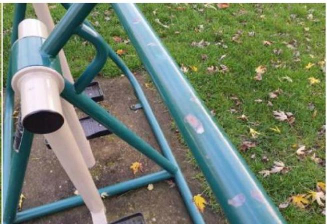
**Finding:** The paintwork on this item has been damaged or worn exposing the metal underneath which is rusting      **Action:** Treat any rusting components and repaint
