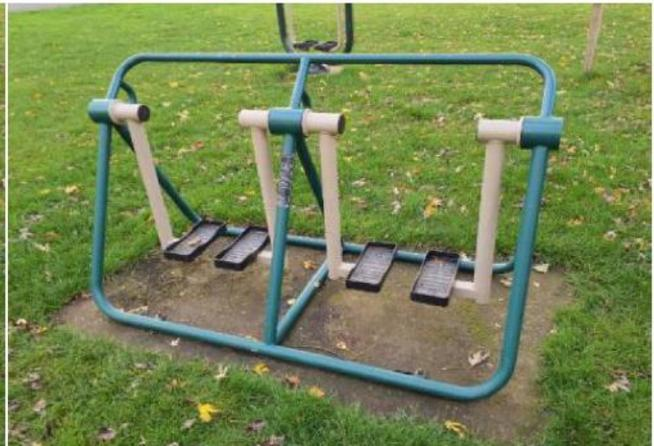
**Finding:** This fitness equipment has been scaled down and is not covered by the scope of BS EN 16630 which specifically relates to equipment for users of 140cm and above. We have however used our knowledge of this standard to form the basis of our assessment as it is the closest applicable standard available
