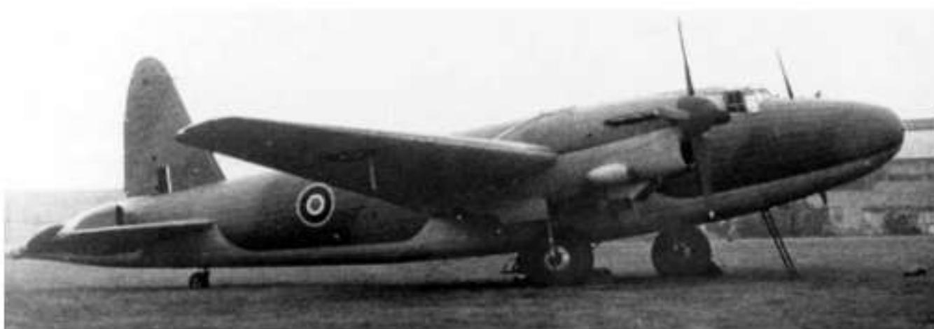
Wellington test beds W5389G and Z8570G - NAM archives Balderton had been chosen because it had concrete runways which were unaffected by the blast from the jet engines, a smoother take off run – there had been some tailwheel collapses due to the extra weight taking off from the grass airfield at Hucknall - and there were no RAF units stationed there at the time.
